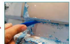
This is useful too: use the rounded tip for scraping off adhesive and small pieces when removing .
